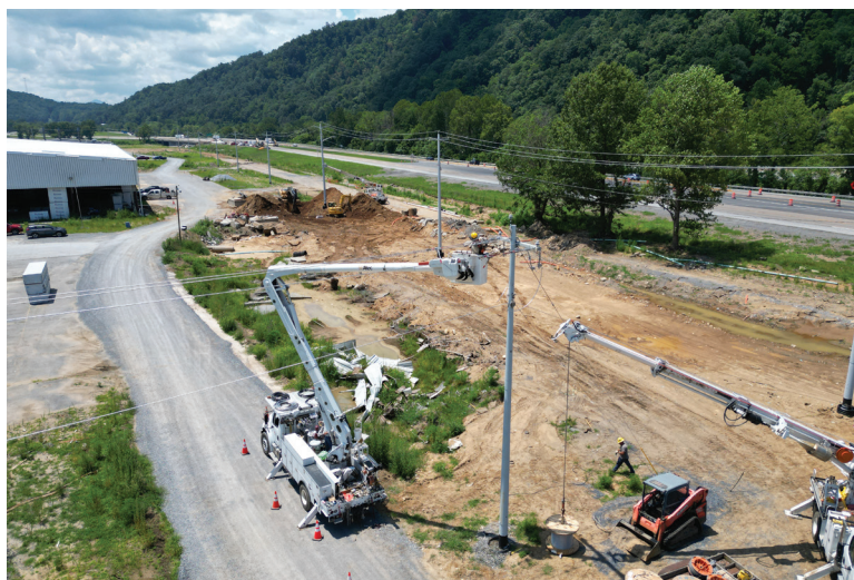
New poles and distribution lines were installed in the Riverview Industrial Park following the extensive damage from Hurricane Helene.
