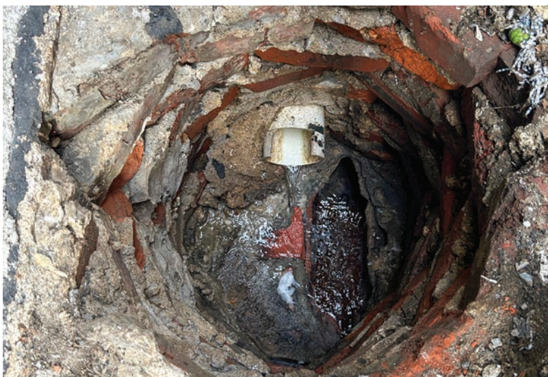
Part of the sewer infrastructure program includes rehabilitating the manholes, above right. Once repaired, above left, crews will rehabilitate the failed lateral to resume proper flow.
